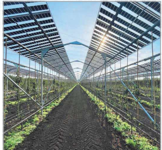
Trellex RE supplies the materials for building solar panels over fruit. Trellex
